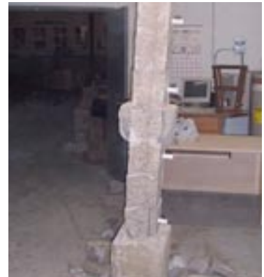
Figure 11: Post Core After Testing and Demolition
